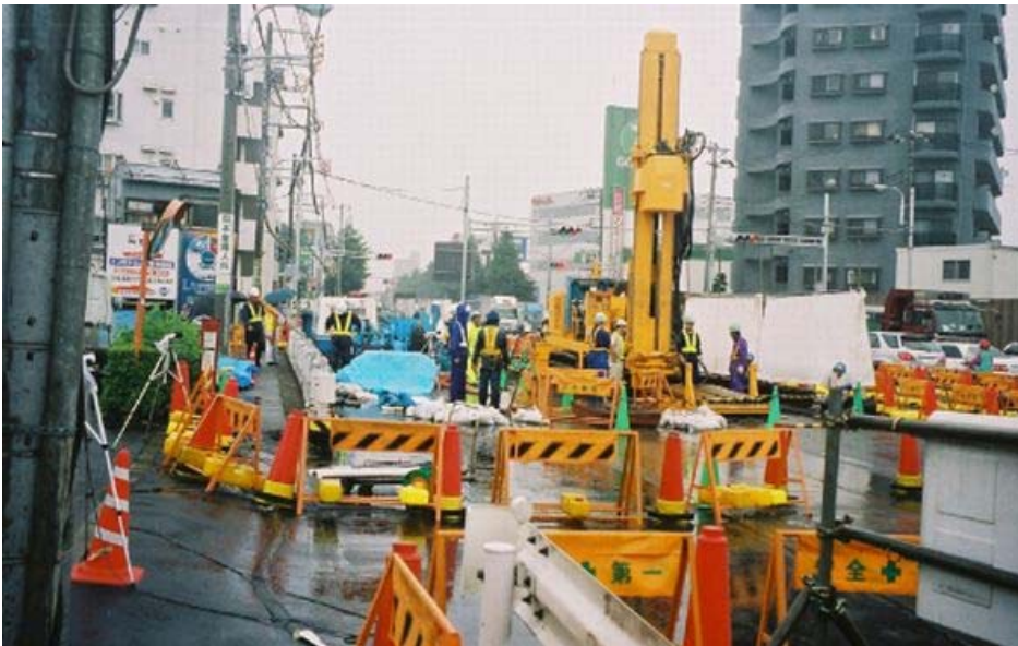
A recent demonstration of sonic drilling in Tokyo, Japan.
