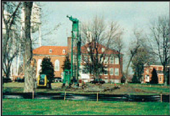
Fort Knox, KY, Creating Bore holes for GSHP
