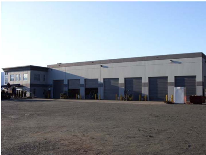
View of Sonic Drill Corp.'s seven easy access equipment bays.
